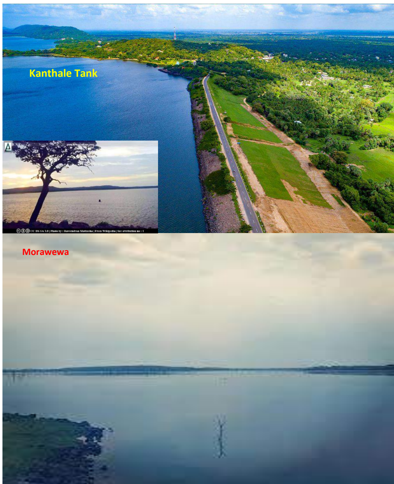
Figure 23: Tanks in Trincomalee District
