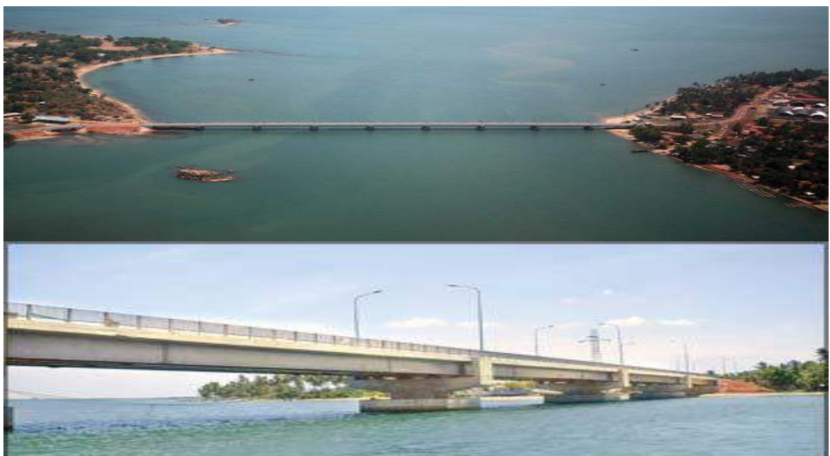
Figure : 27 Trincomalee – Kinniya Bridge
