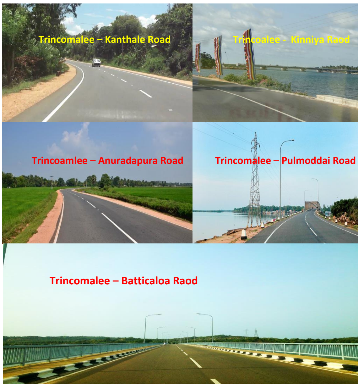
Figure 26: Roads in Trincomalee
