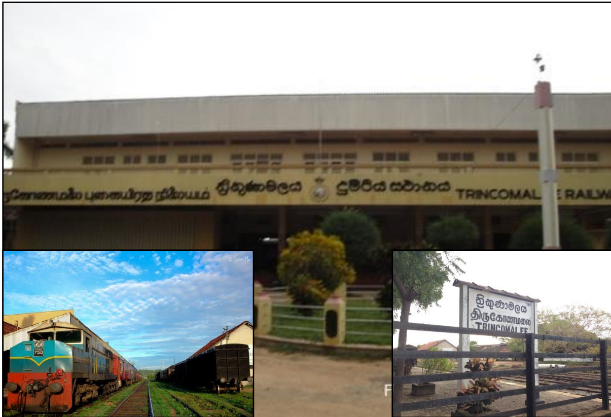
Figure : 29 Trincomalee Railway Station
