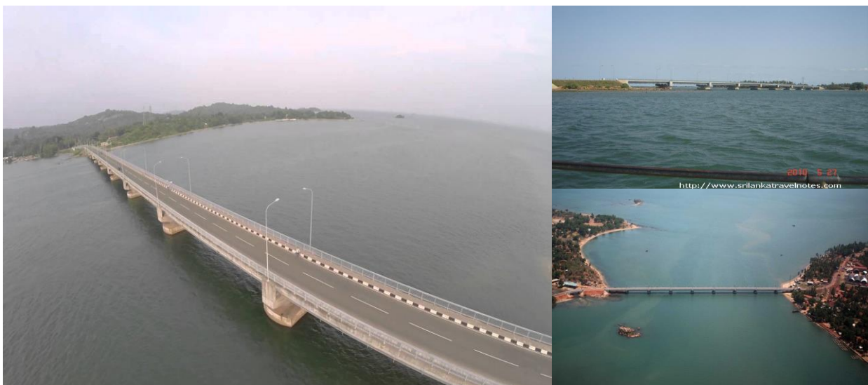
Figure : 27 Trincomalee – Kinniya Bridge
